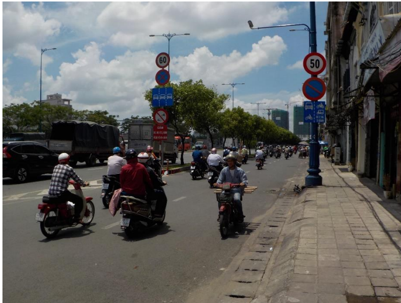
Photo 11. Separation of motorcycles from other motorized vehicles by means of a dedicated motorcycle lane in Viet Nam
