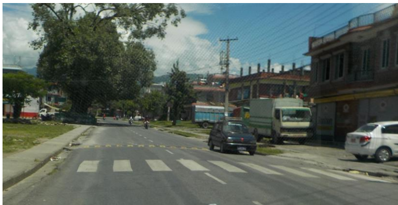
Photo 6. Example of speed hump on approach to pedestrian crossing in Nepal.
