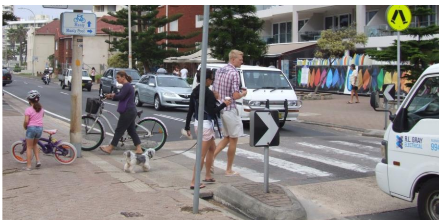
Photo 7. Example of raised platform crossing in Australia.
