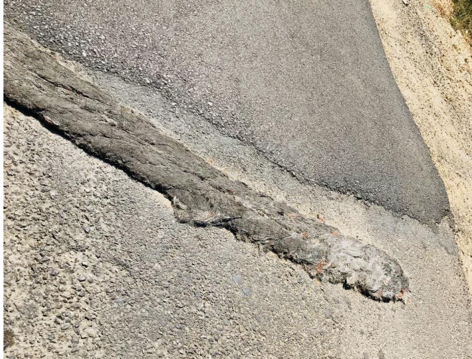
Photo 5. Example of a community-created speed hump, indicating that people want lower speeds in their community.
